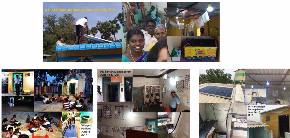
Figure 3: First four PV systems installed at village Single Teacher Schools, Tamil Nadu 2017
